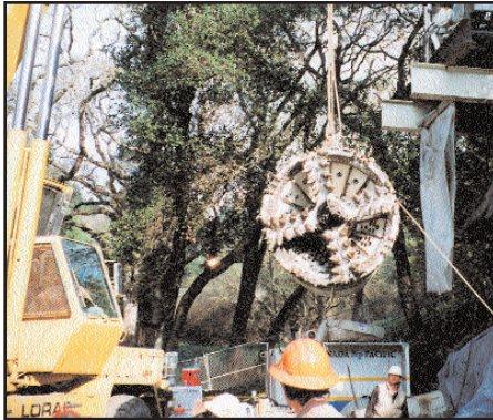
Top: Nada Pacific lowers the 44-in. Akkerman microtunneler into a launch pit.
